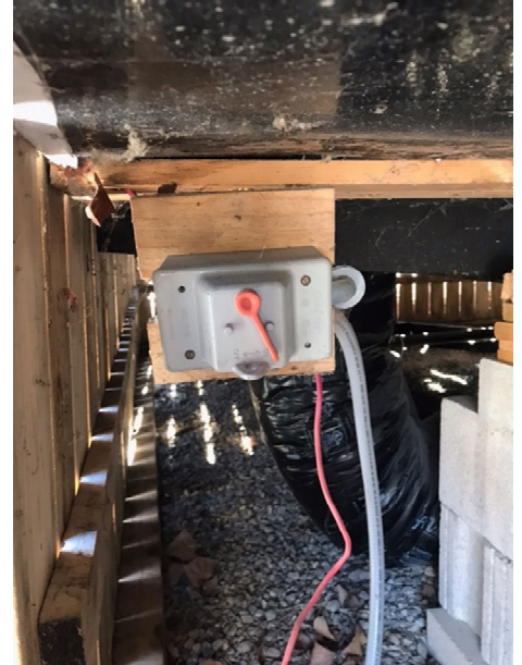
A/C shut off switch on outside of cottage
