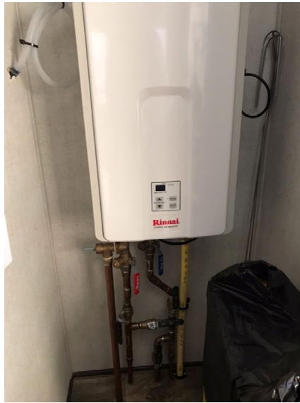
Tankless hot water tank & valves
